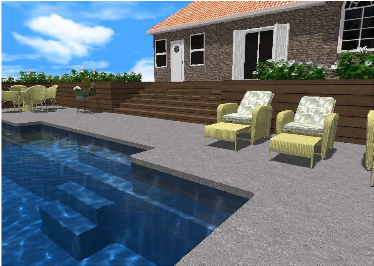
Wood retaining wall built of 6x6 pressure treated lumber
